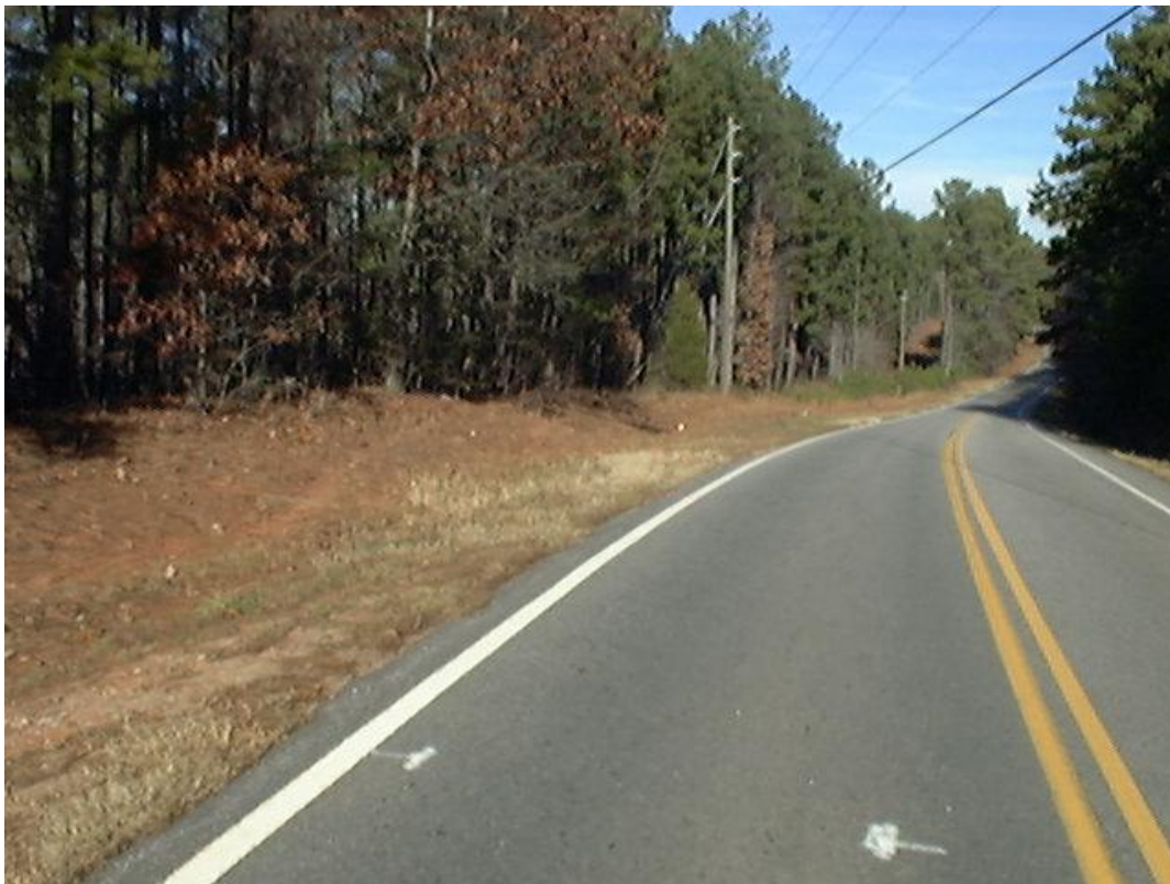
General view of the accident scene showing departure from road
