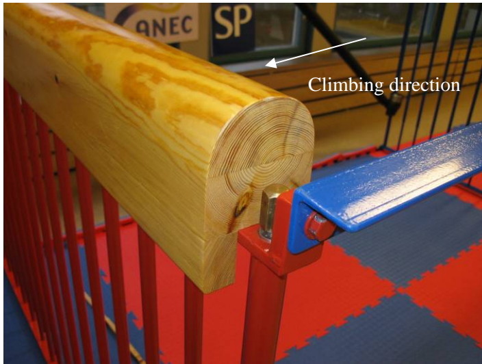
Photo 2.5. 100 mm wide top profile mounted on the barrier.
